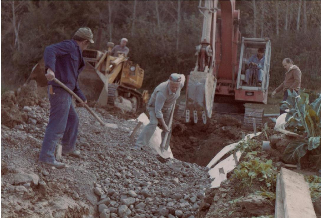
*Drainage trenches along slopes (4/7 meters deep) with bottom pipe, non-woven fabric and drainage material*
