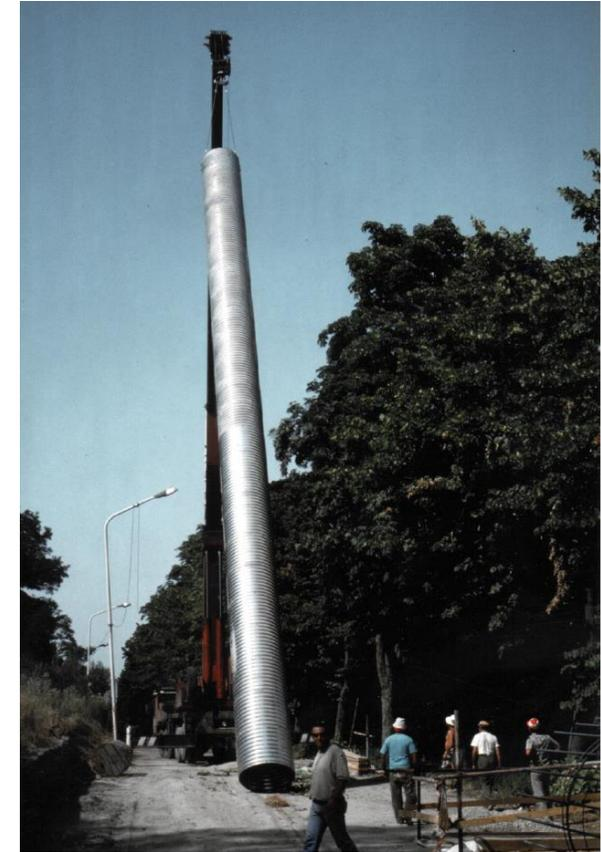
*Small-diameter drainage wells with bottom pipeline*
