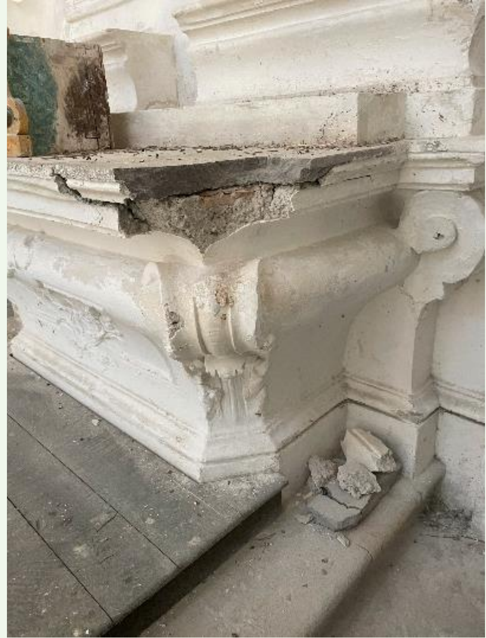
Rainwater infiltrations and cracking of stuccos
