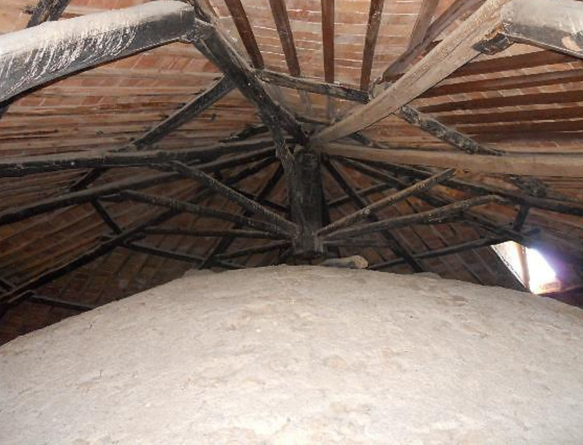
The circular truss that supports the roof above the dome: very dangerous situation especially due to the limited size of the wooden elements
