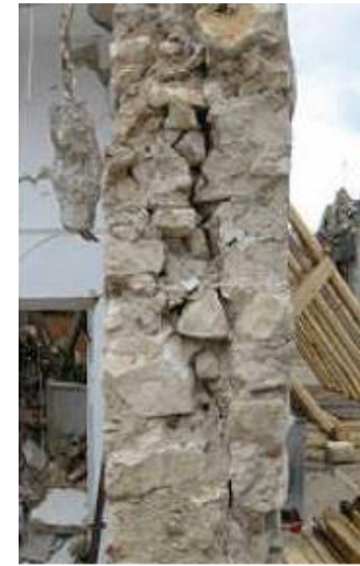
THE DISINTEGRATION MECHANISM OF MASONRY
