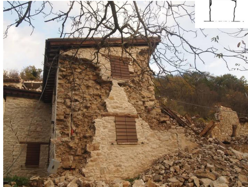
THE DISINTEGRATION MECHANISM OF MASONRY
