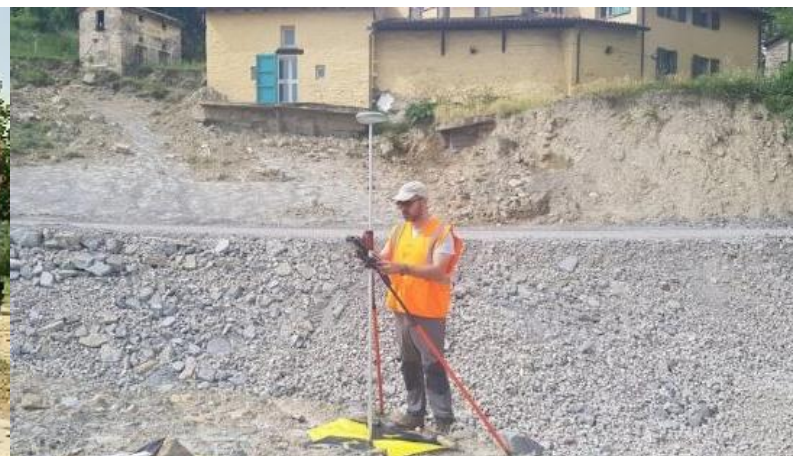
GNSS Survey on Ground Control Point (GCP)
