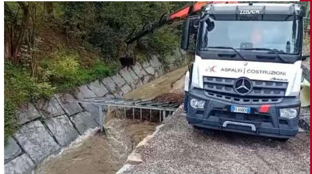
18/09/2024 - Cleaning up from debris deposited from previous floods on the Ravone stream
