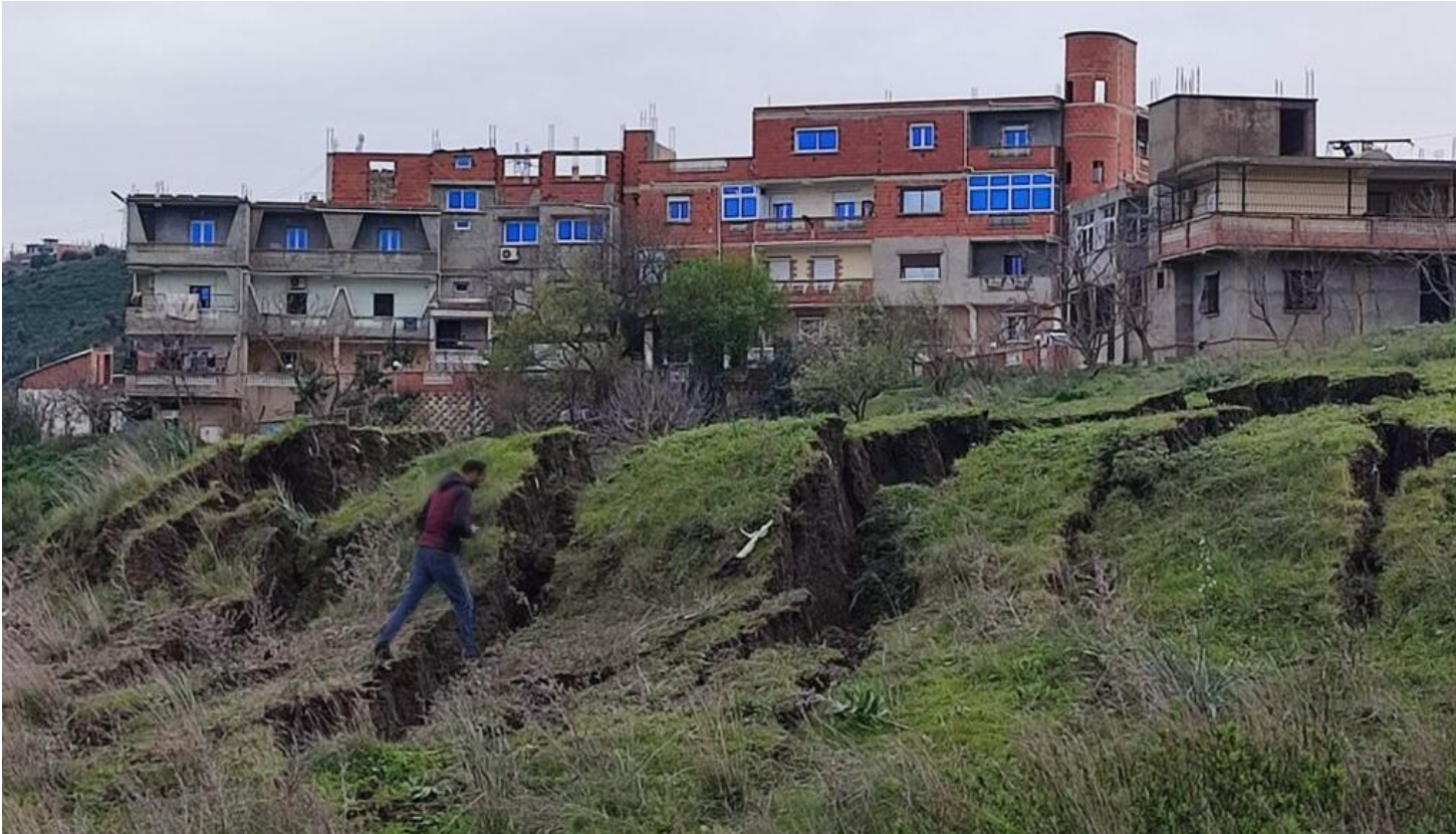
Ground cracking and slope deformation near dwellings — public Facebook/local photo post, 27 Feb. 2025.
