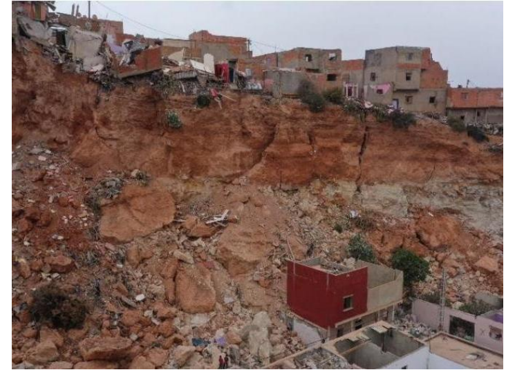
Visible scar and exposed landslide front
