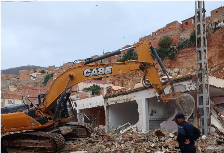
Demolition and exposure reduction after evacuation
