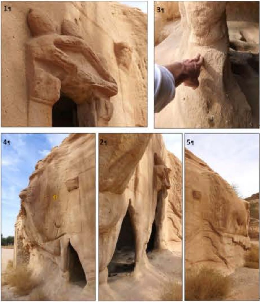
Fig 3: Details of geomorphological phenomena: Centimetre exfoliation of the ceiling and erosion of the pillars; deep basal erosion
