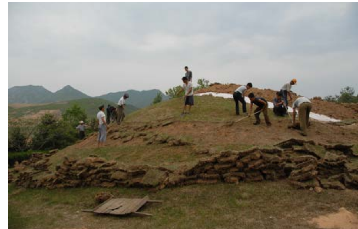
Waterproofing the tombs
