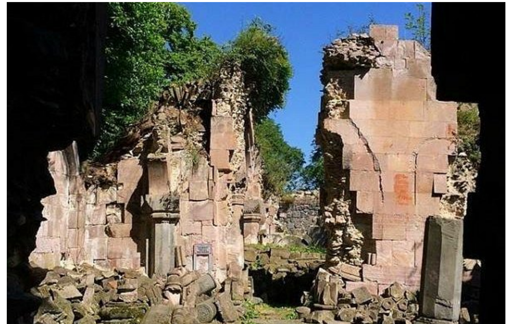
Likely earthquake-induced landslide in Bardzrakash, Armenia
