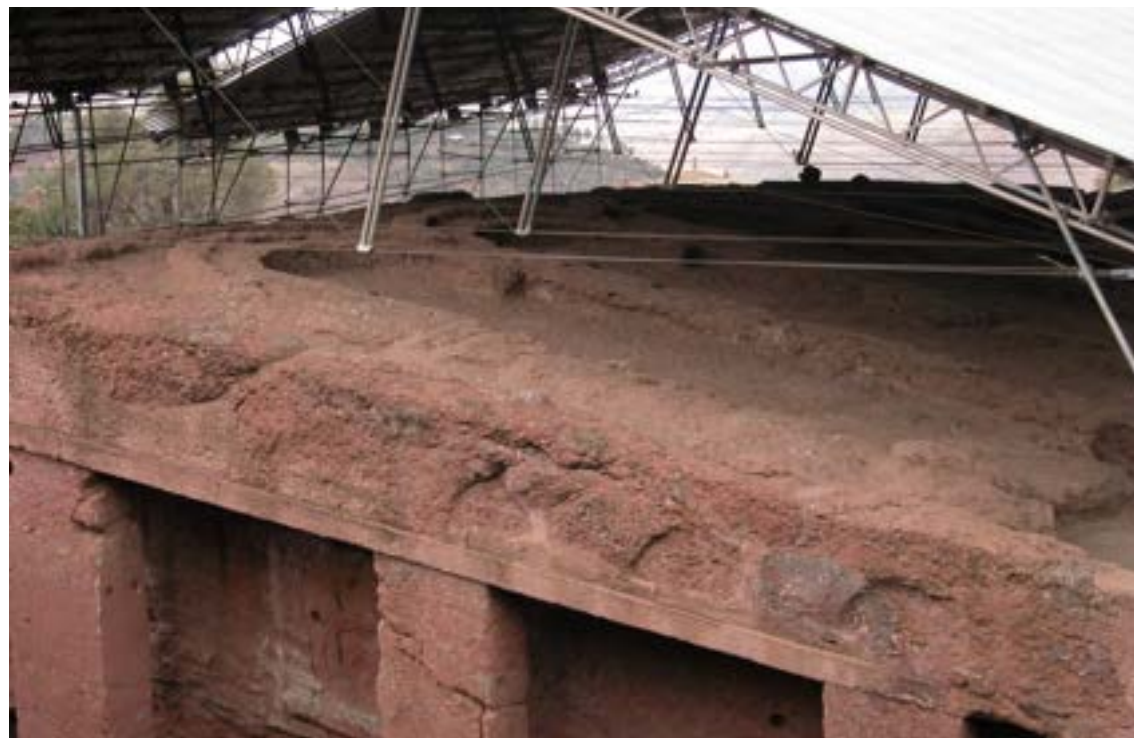
Example: weathering of the roof
