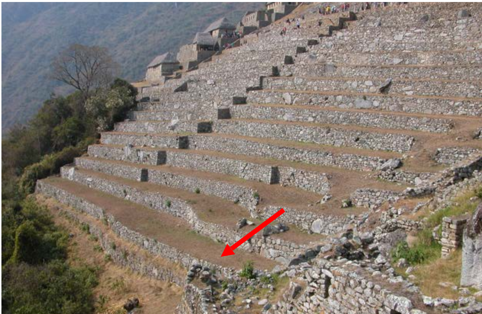
Earth slide deforming the andenas of Machu Picchu - Peru
